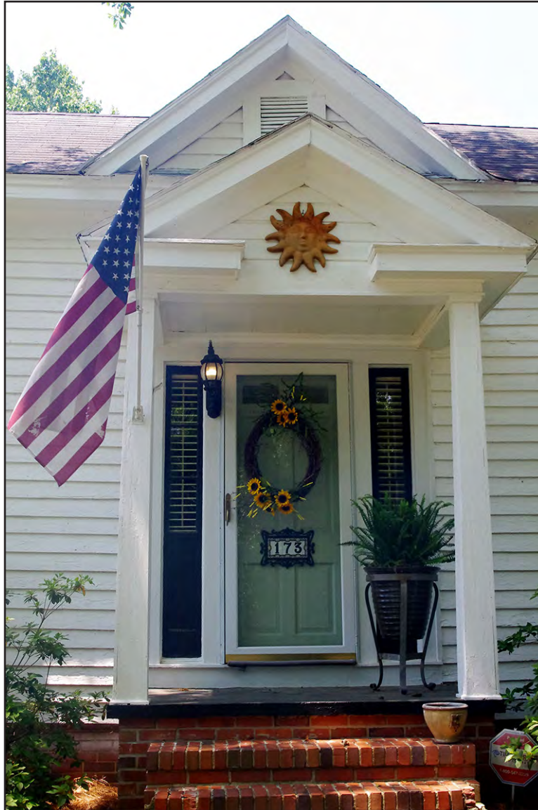
PLATE 111: Detail of Main Entrance on East Elevation, Gibson-McDonald House (RH0156), Rockingham, North Carolina
