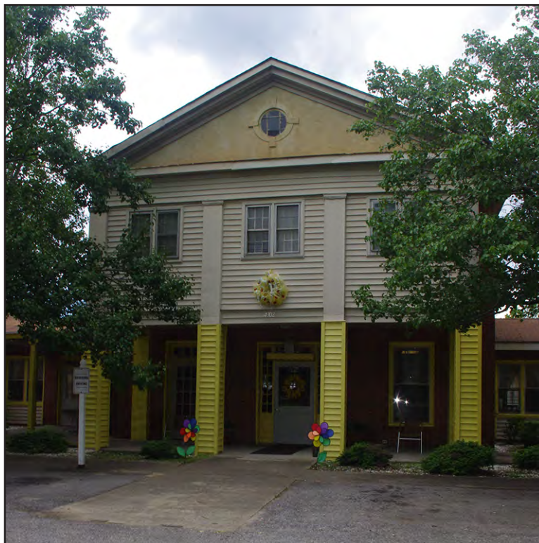
PLATE 30: Former Johnston County Home (JT0825), South Elevation of Main Block, Johnston County, North Carolina
