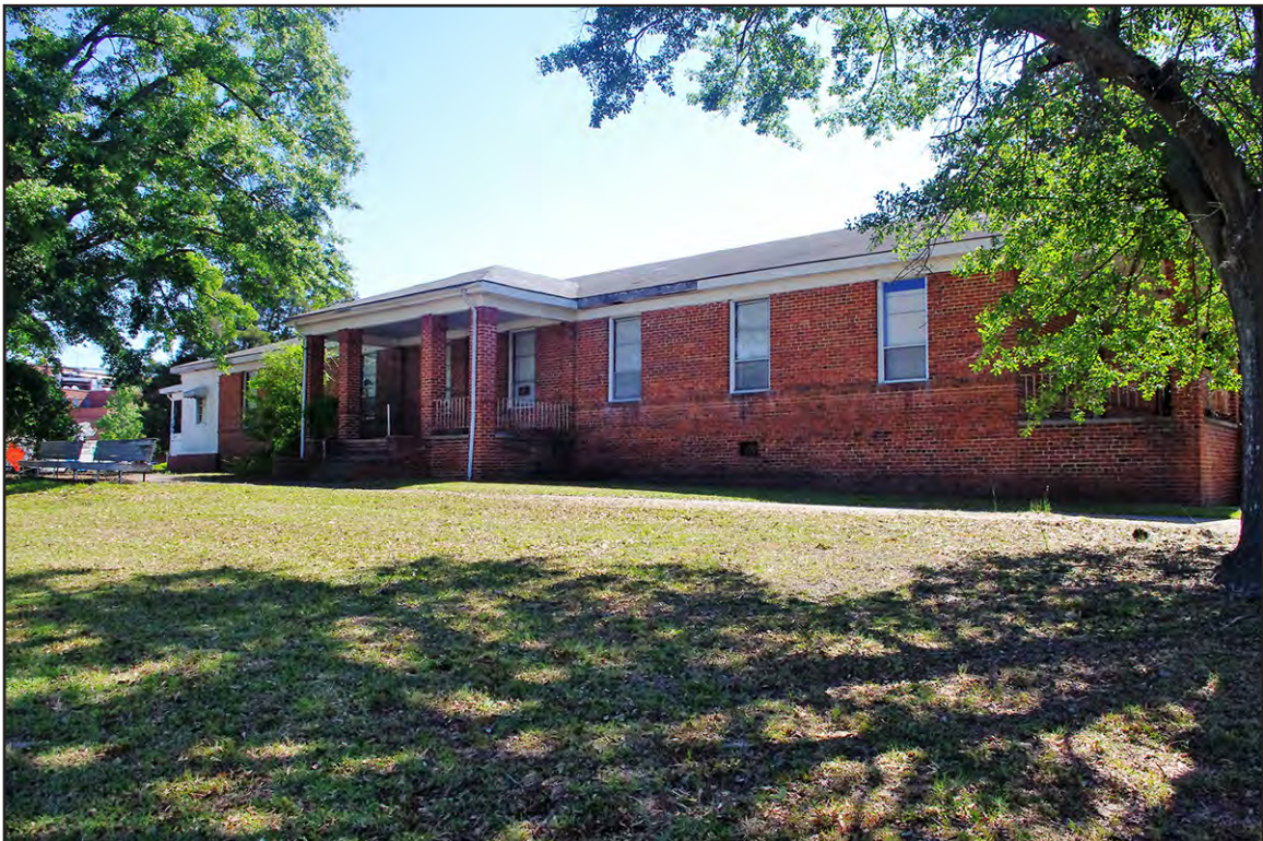
PLATE 18: Glenwood Rest Home (County Home) (RH0667), West elevation of Far Western Wing, Rockingham, North Carolina
