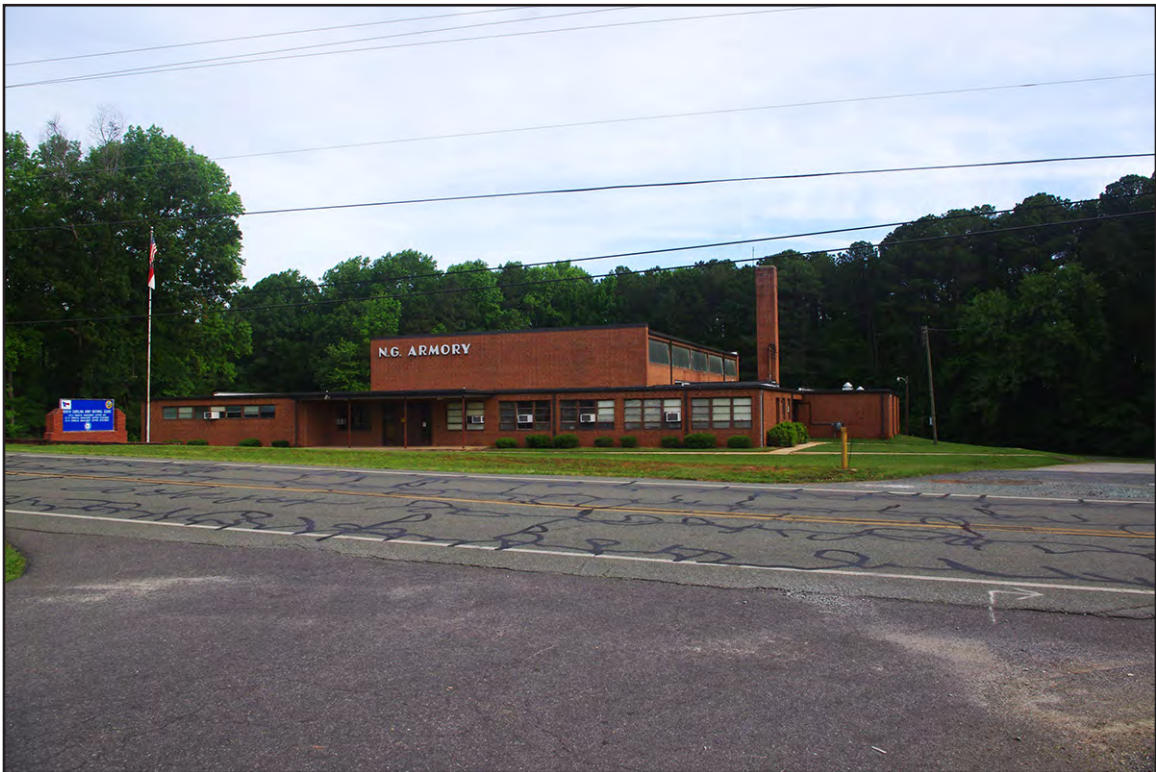
PLATE 9: Siler City National Guard Armory (CH0819), South Elevation, Chatham County, North Carolina
