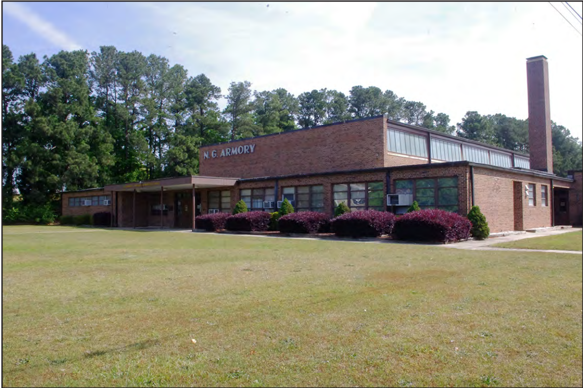
PLATE 1: Rockingham National Guard Armory (RH0737), West and South Elevations, Rockingham, North Carolina
