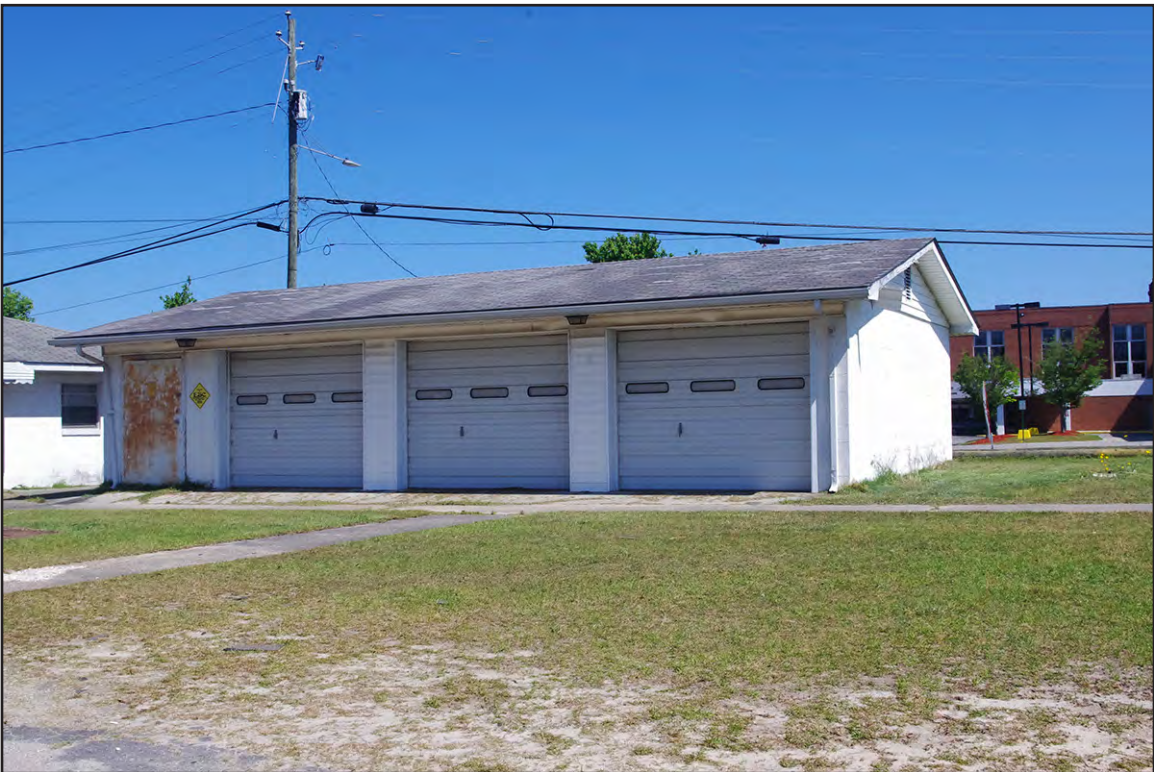
PLATE 25: Garage North of the Richmond County Home (RH0667), South Elevation, Rockingham, North Carolina
