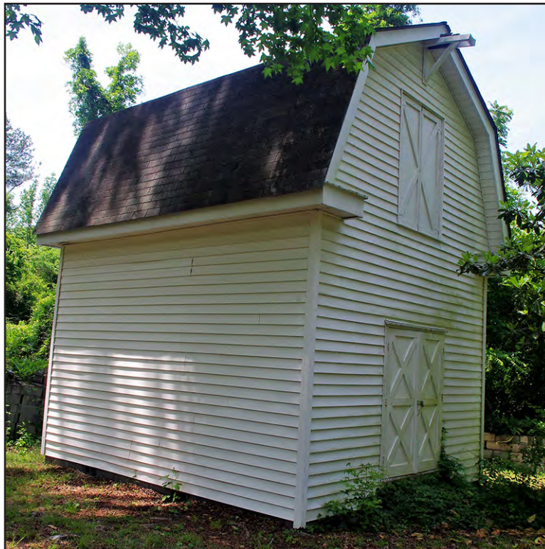
PLATE 92: Shed, North and East Elevations, Elliot-Terry-Mossor Farm (RH0297), Rockingham, North Carolina
