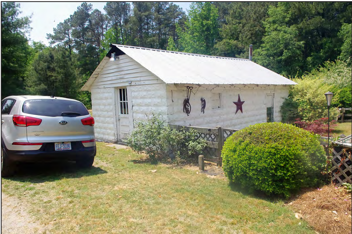
PLATE 116: Storage Outbuilding, North and East Elevations, Gibson-McDonald House (RH0156), Rockingham, North Carolina
