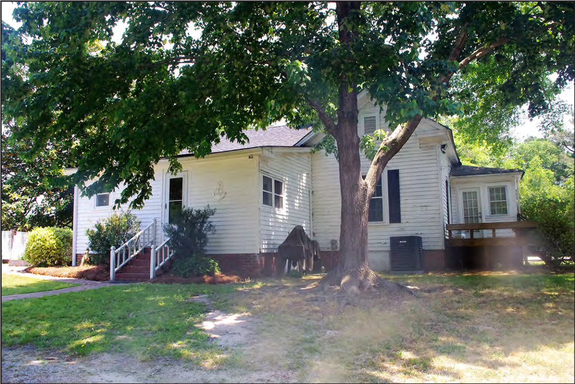
PLATE 113: Gibson-McDonald House (RH0156), West Elevation, Rockingham, North Carolina
