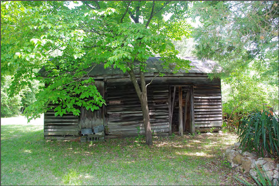
PLATE 89: Cook/Help House, South Elevation, Elliot-Terry-Mossor Farm (RH0297), Rockingham, North Carolina
