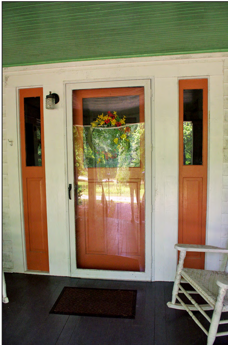
PLATE 73: Detail of Main Entrance on East Elevation, Elliot-Terry-Mossor House (RH0297), Rockingham, North Carolina
