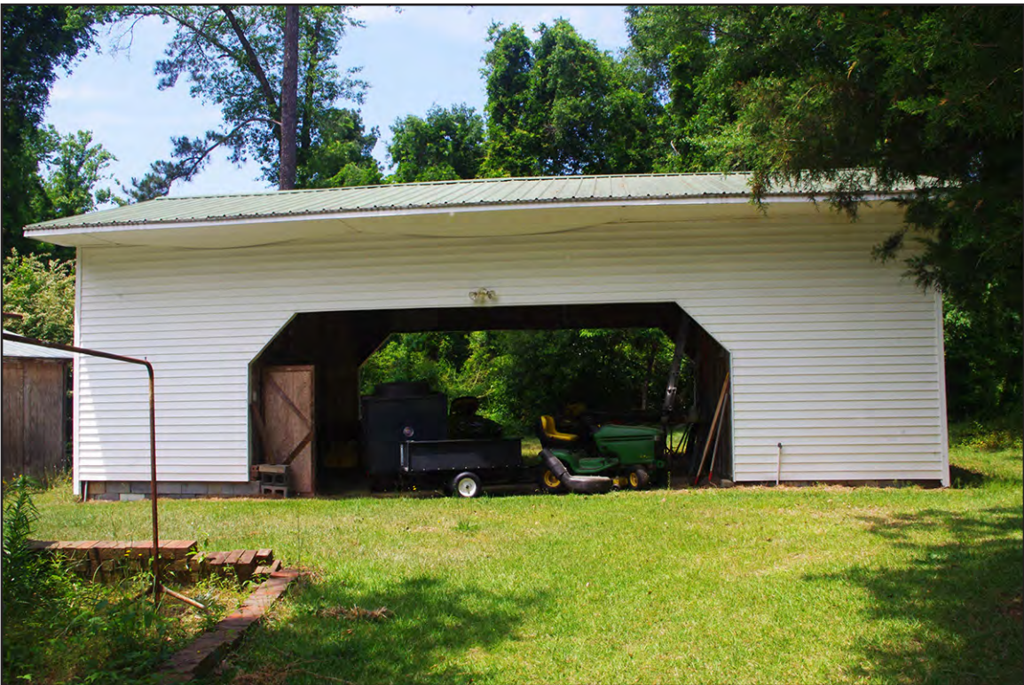
PLATE 88: Large Storage Barn, East Elevation, Elliot-Terry-Mossor Farm (RH0297), Rockingham, North Carolina
