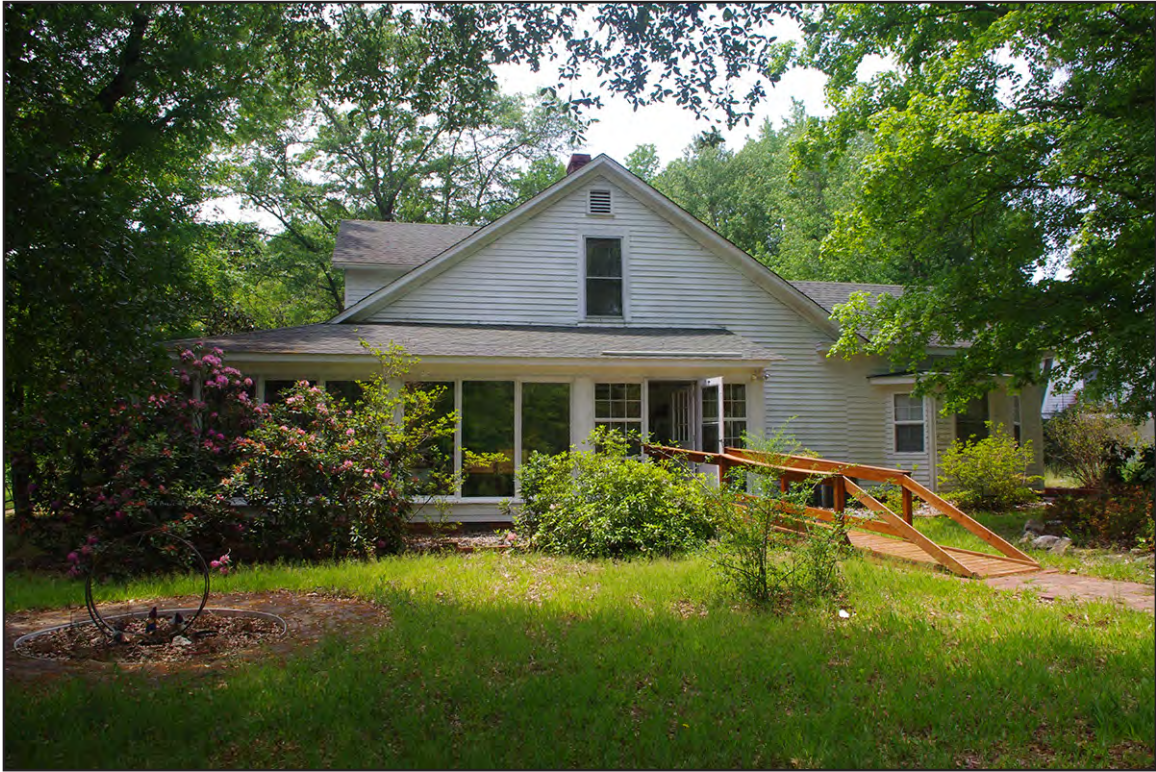
PLATE 71: Elliot-Terry-Mossor House (RH0297), North Elevation, Rockingham, North Carolina
