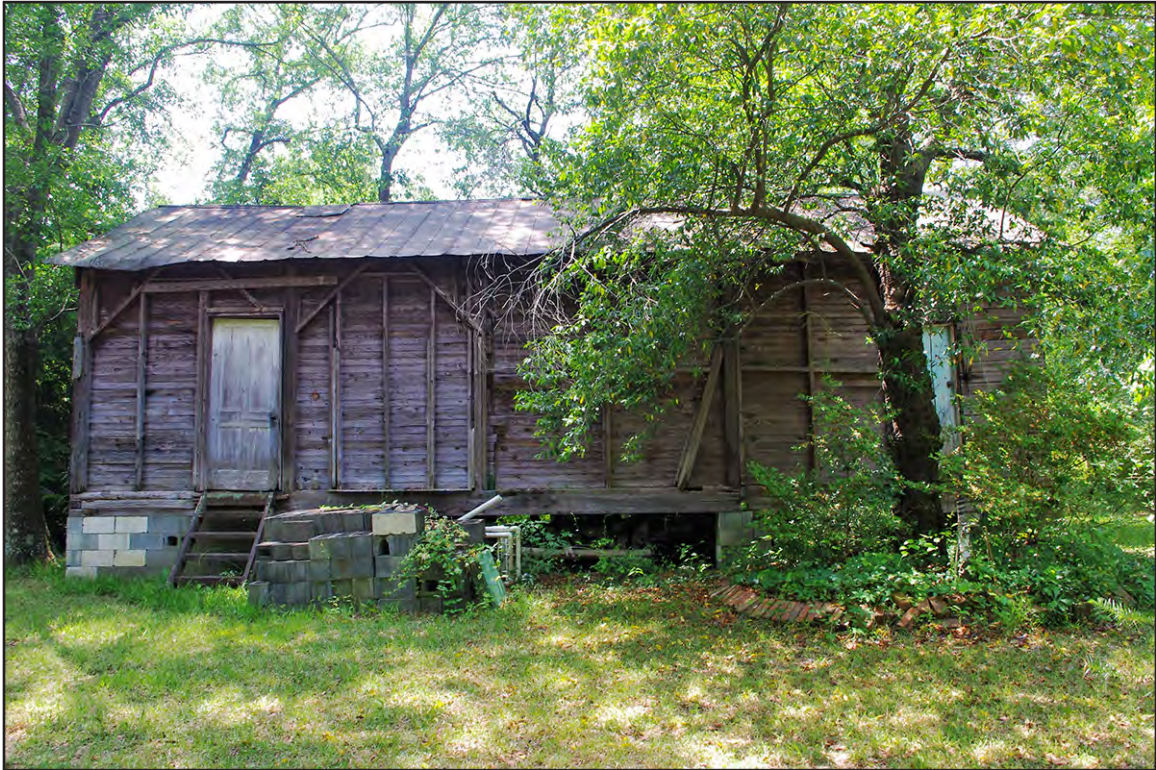
PLATE 80: Terry Store, North Elevation, Elliot-Terry-Mossor Farm (RH0297), Rockingham, North Carolina
