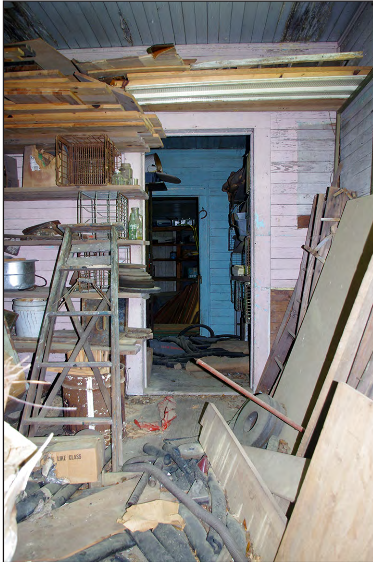
PLATE 82: Interior of Terry Store, Looking East, Elliot-Terry-Mossor Farm (RH0297), Rockingham, North Carolina
