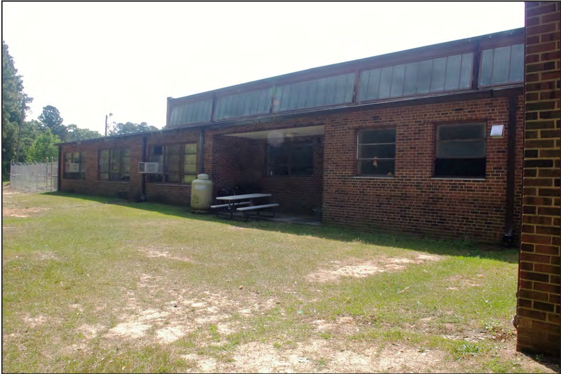
PLATE 3: Rockingham National Guard Armory (RH0737), North Elevation, Rockingham, North Carolina
