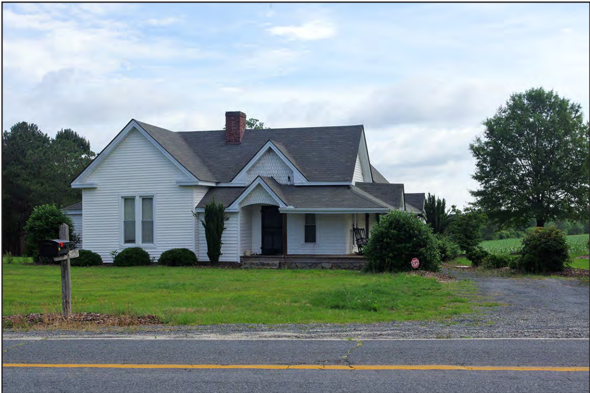
PLATE 119: Lentz House (RH0449), South Elevation, Richmond County, North Carolina
