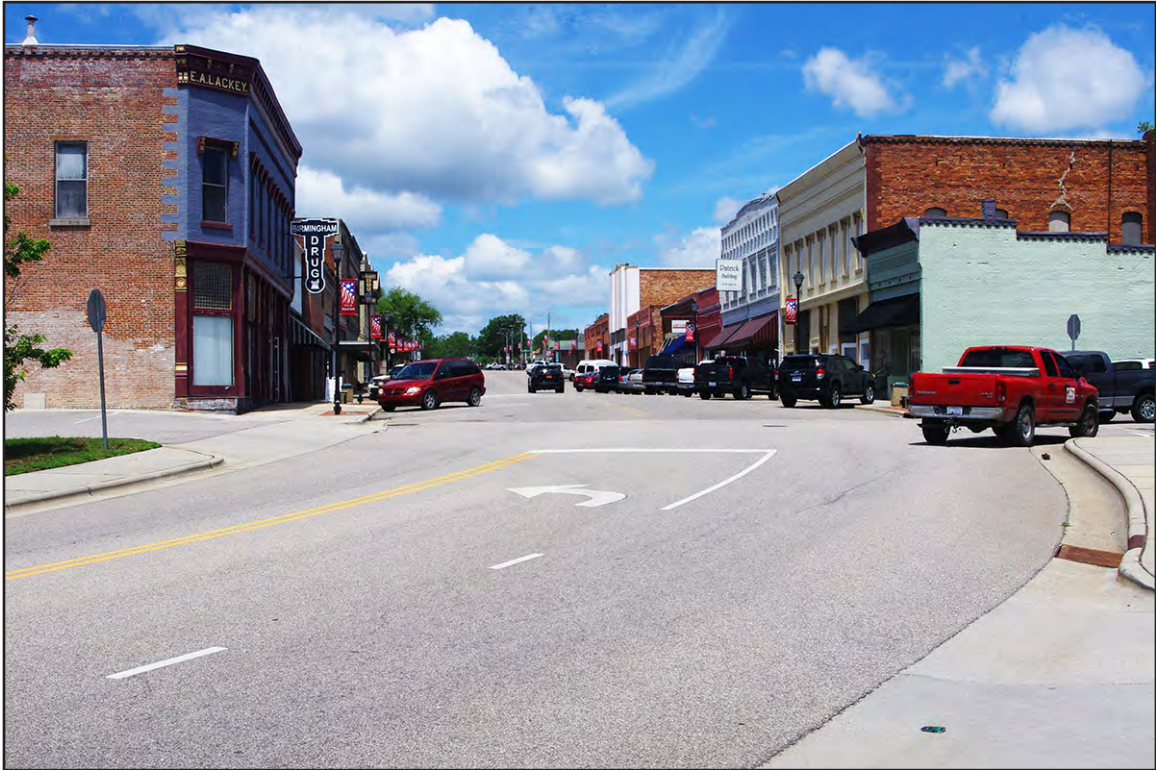
PLATE 44: Looking North on Main Street, Main Street Commercial District (RH0010), Hamlet, Richmond County, North Carolina
