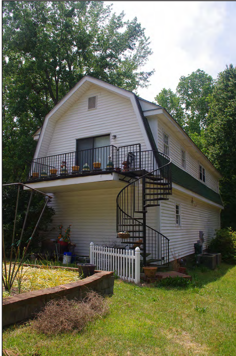
PLATE 79: Carriage House, North Elevation, Elliot-Terry-Mossor Farm (RH0297), Rockingham, North Carolina
