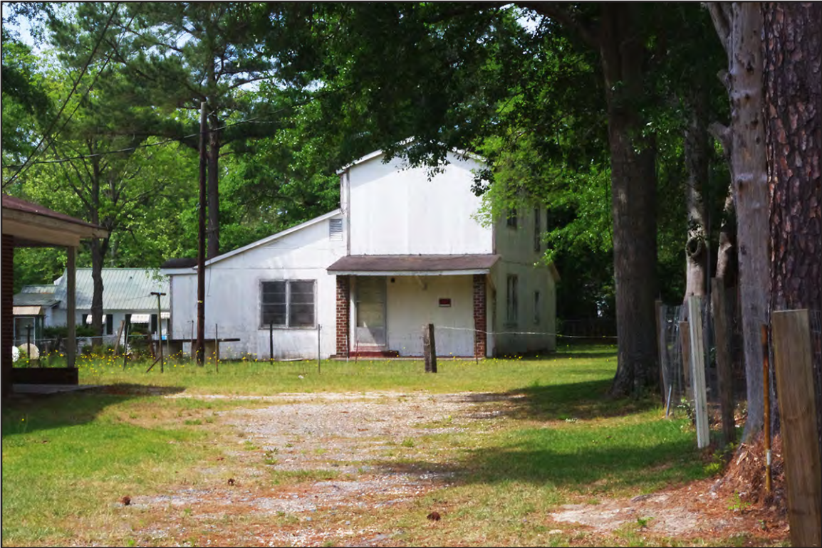
PLATE 64: Unidentified Building No. 1 on J.E. Haywood House Property, North Elevation, Rockingham, North Carolina
