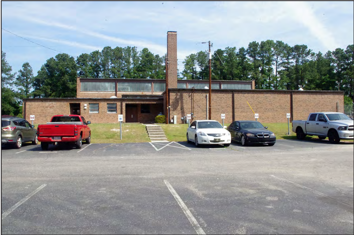
PLATE 5: Rockingham National Guard Armory (RH0737), South Elevation, Rockingham, North Carolina
