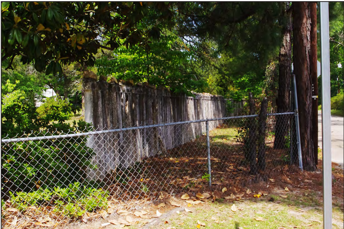
PLATE 60: Concrete Fence on Former J.E. Haywood House Property, Looking East, Rockingham, North Carolina
