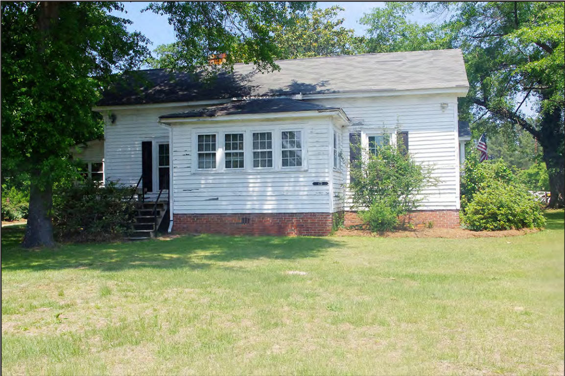
PLATE 112: Gibson-McDonald House (RH0156), South Elevation, Rockingham, North Carolina
