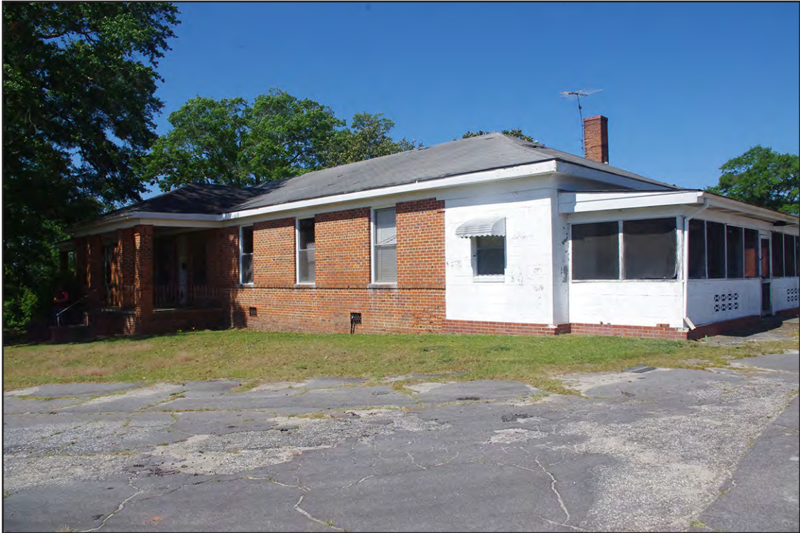
PLATE 33: Glenwood Rest Home (County Home) (RH0667), East Elevation of Eastern Wing, Rockingham, North Carolina
