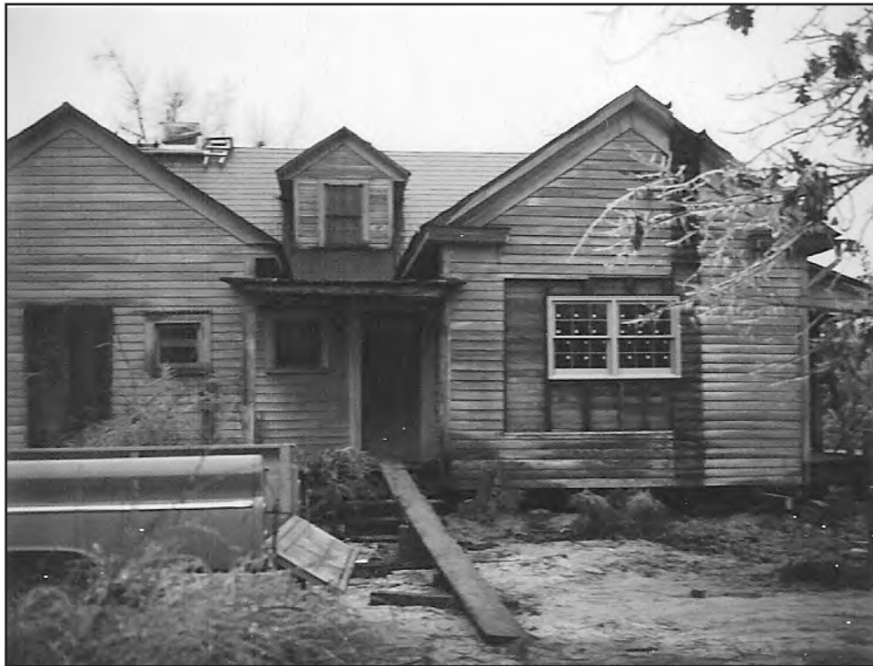
PLATE 102: West Elevation of Elliot-Terry-Mossor House (RH0297) During 1970 Renovation, Rockingham, North Carolina (Courtesy of Jim Mossor)
