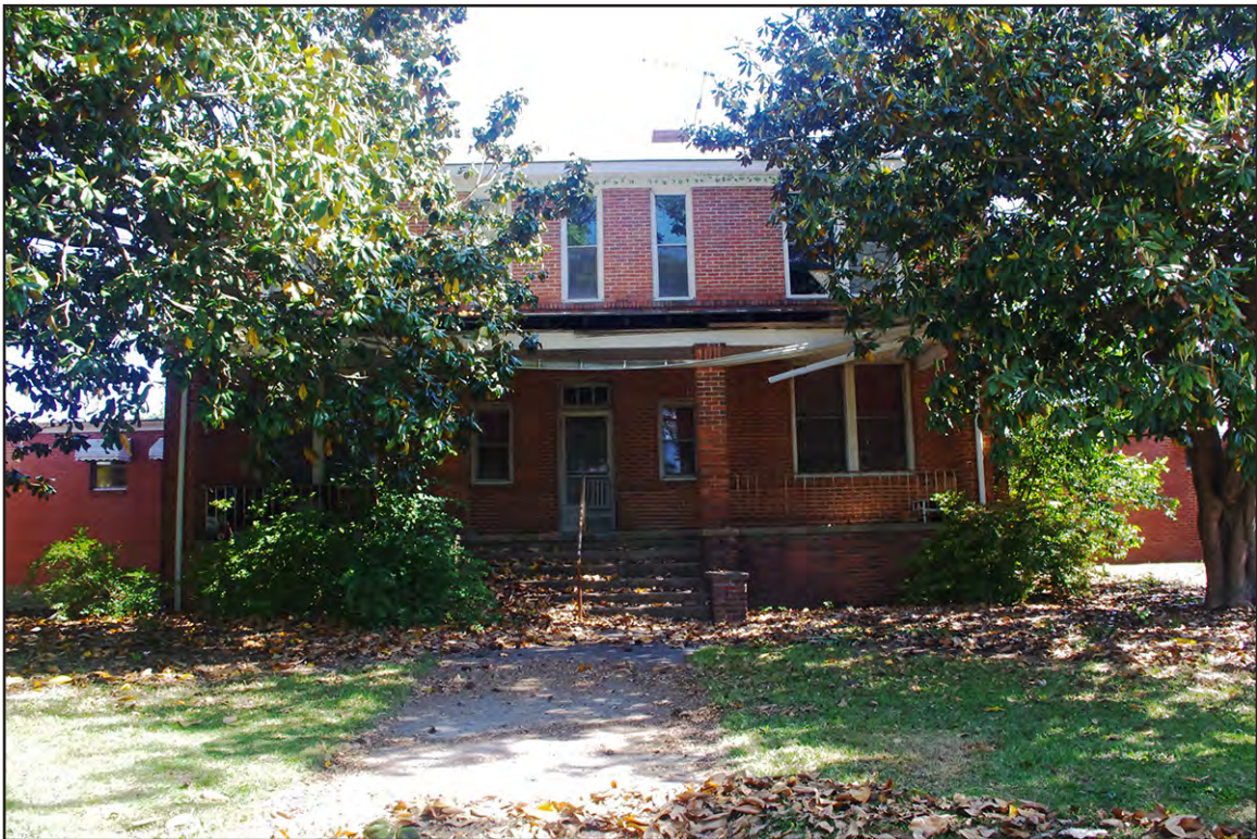
PLATE 12: Glenwood Rest Home (County Home) (RH0667), South Elevation Showing Central Main Block, Rockingham, North Carolina
