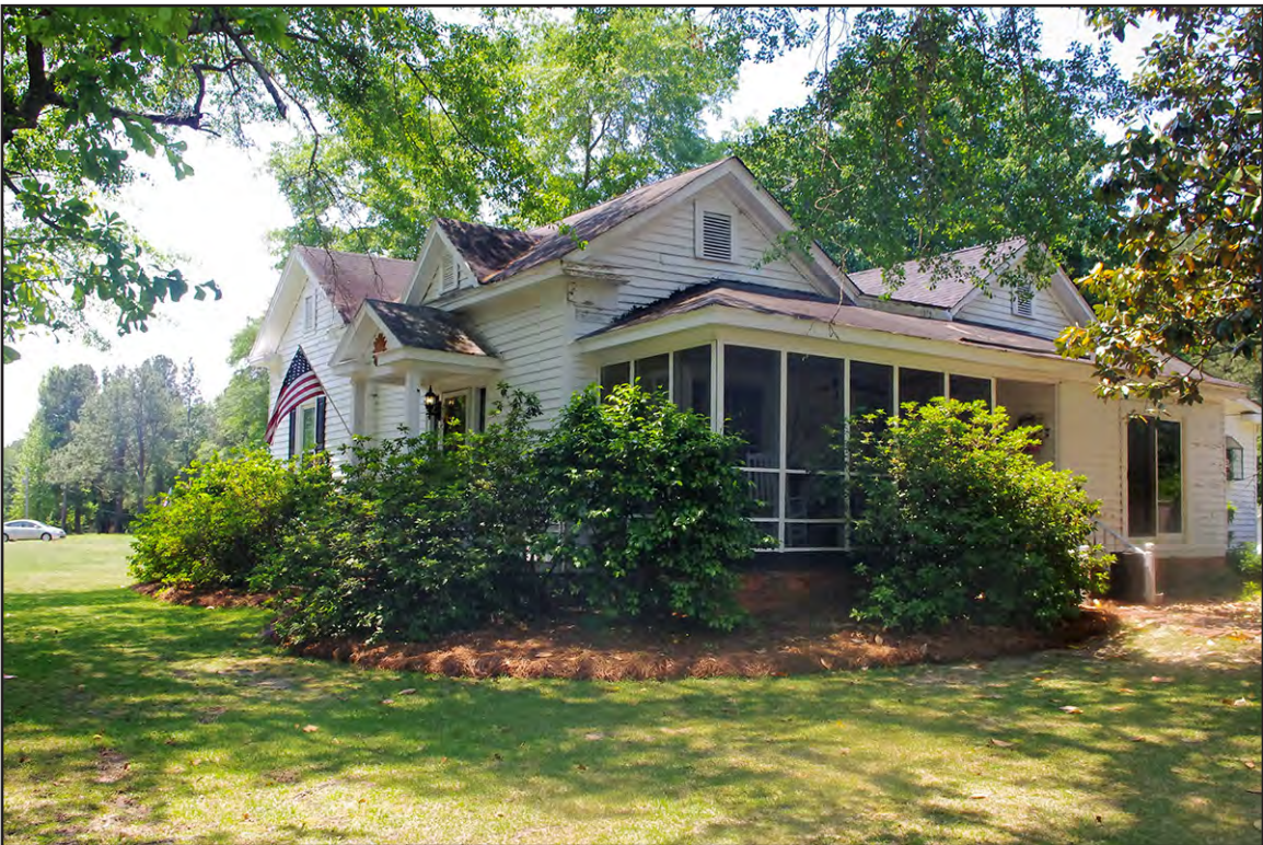
PLATE 114: Gibson-McDonald House (RH0156), North Elevation, Rockingham, North Carolina
