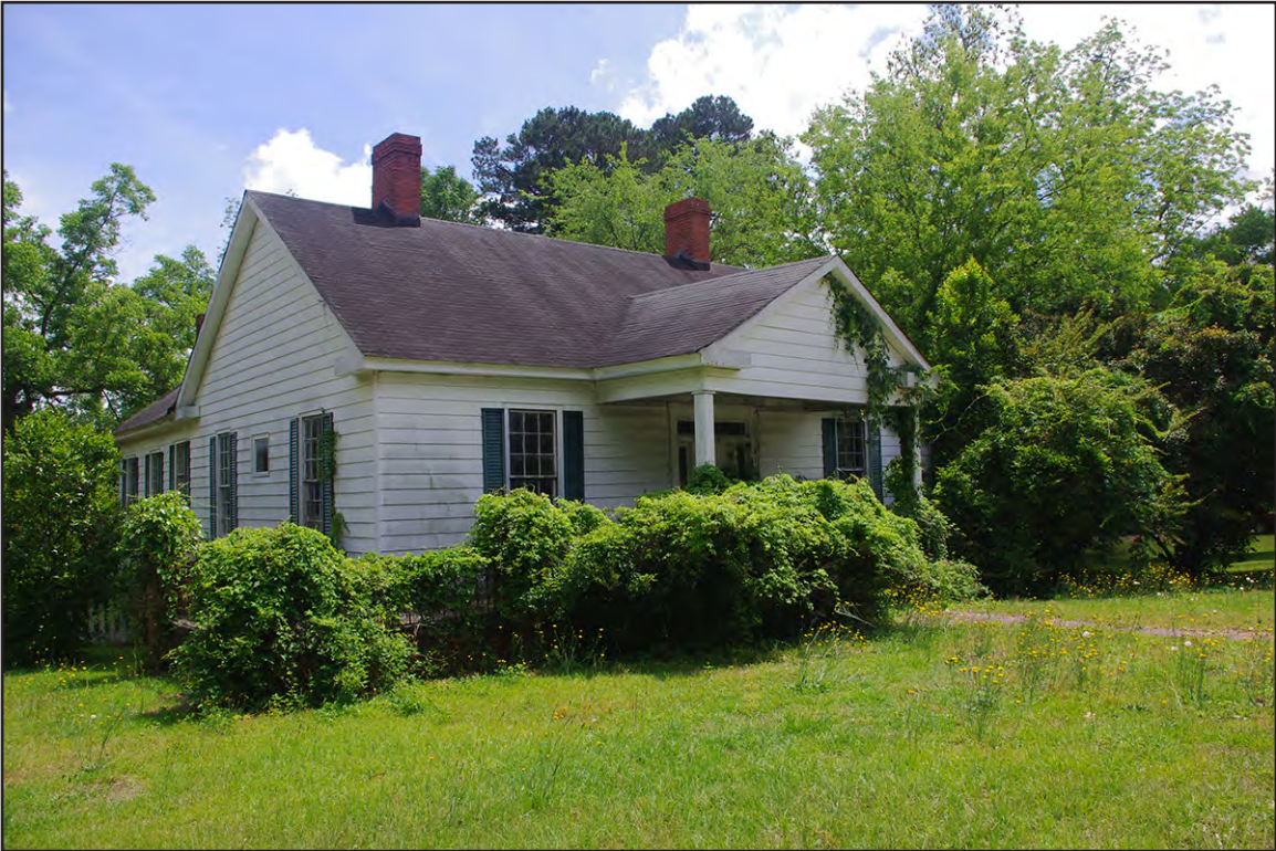
PLATE 122: Stephen W. Steele House (RH0288), North Elevation, Rockingham, North Carolina
