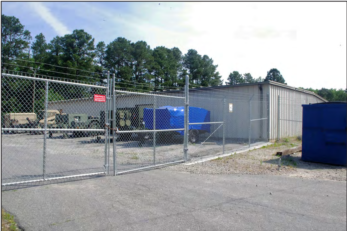
PLATE 7: Rockingham National Guard Armory (RH0737), Motor Pool Area and Workshop, Facing Northeast, Rockingham, North Carolina
