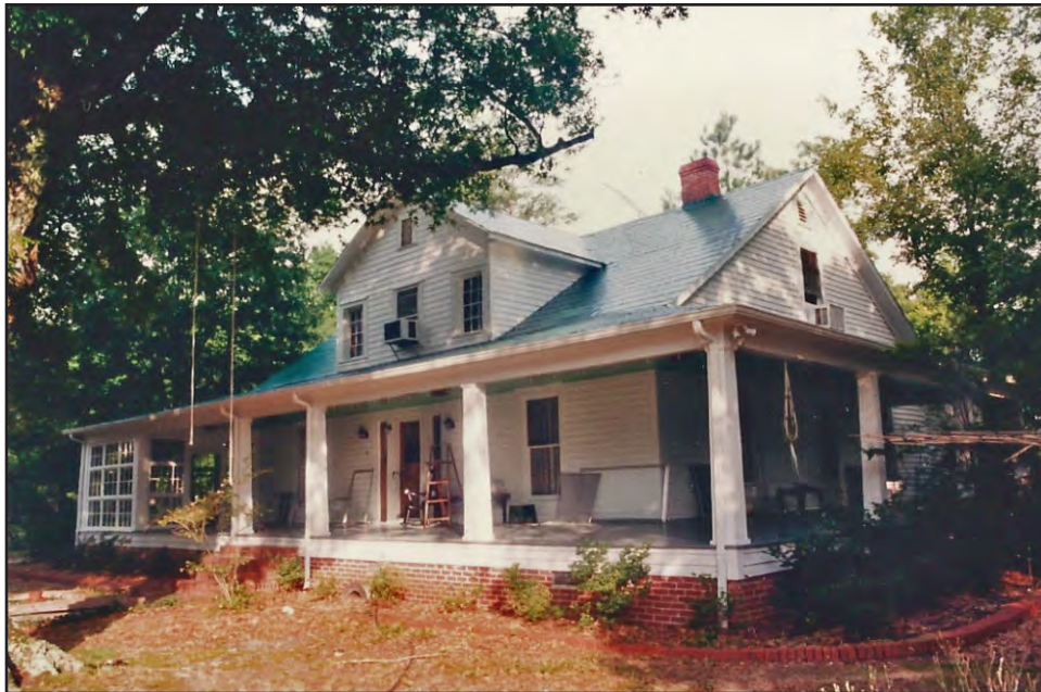
PLATE 108: Elliot-Terry-Mossor House (RH0297), Oblique View of East and North Elevations, Showing Original Open Porch, ca. 1970, Rockingham, North Carolina (Courtesy of Jim Mossor)
