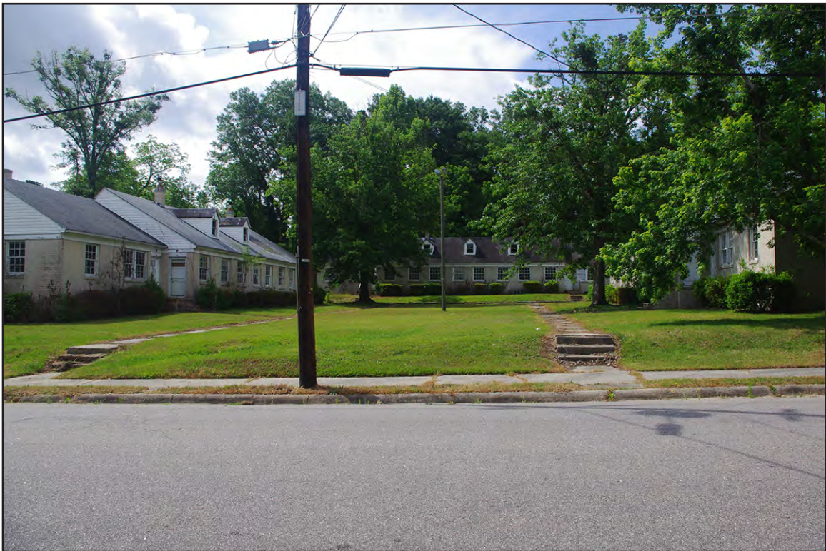
PLATE 38: Apartment Complex, ca. 1930-1940, at Far Western End of Ann Street, Looking South, Rockingham, North Carolina
