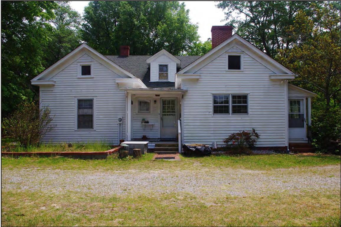
PLATE 74: Elliot-Terry-Mossor House (RH0297), West Elevation, Rockingham, North Carolina
