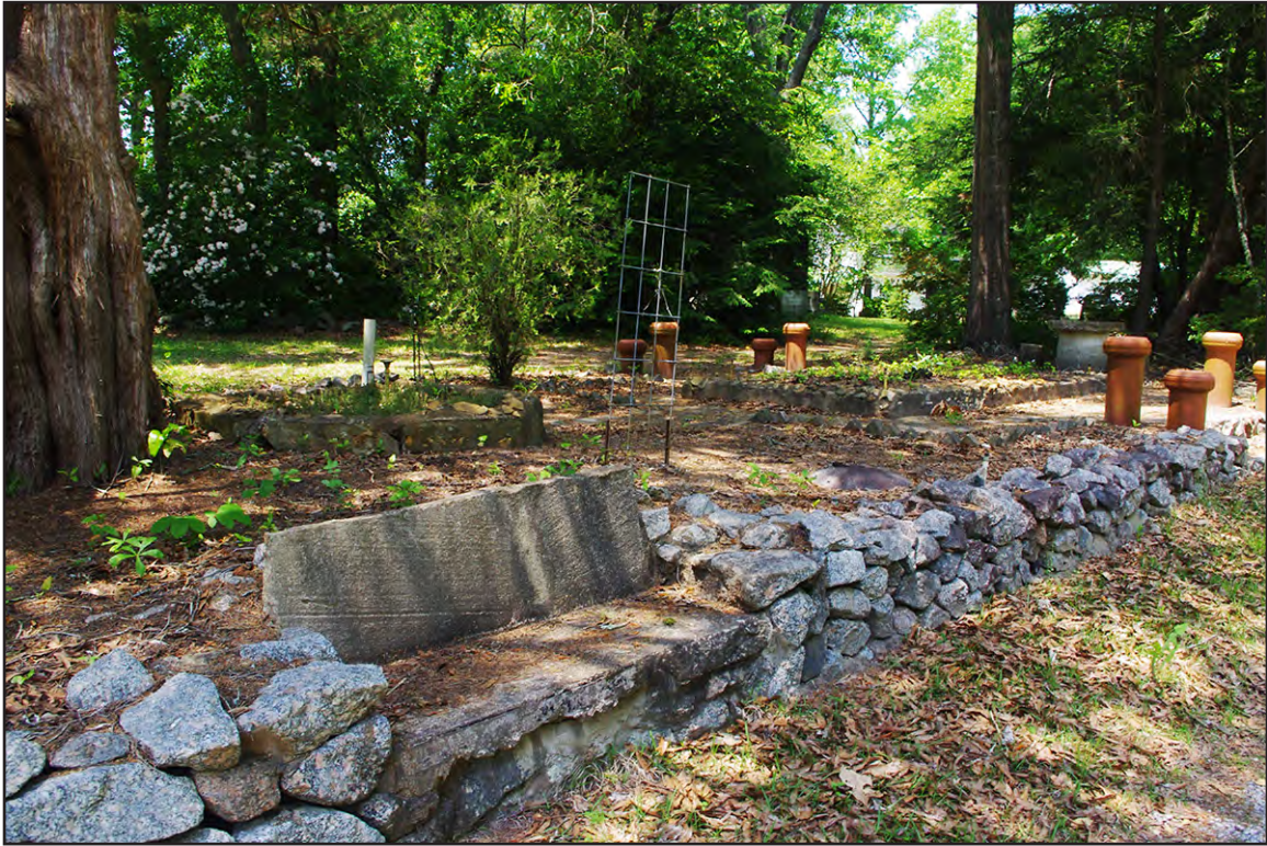
PLATE 69: Rock Wall Containing Landscaped Beds with Built-in Stone Benches Bordering Driveway of Elliot-Terry-Mossor Farm (RH0297), Looking Southwest, Rockingham, North Carolina
