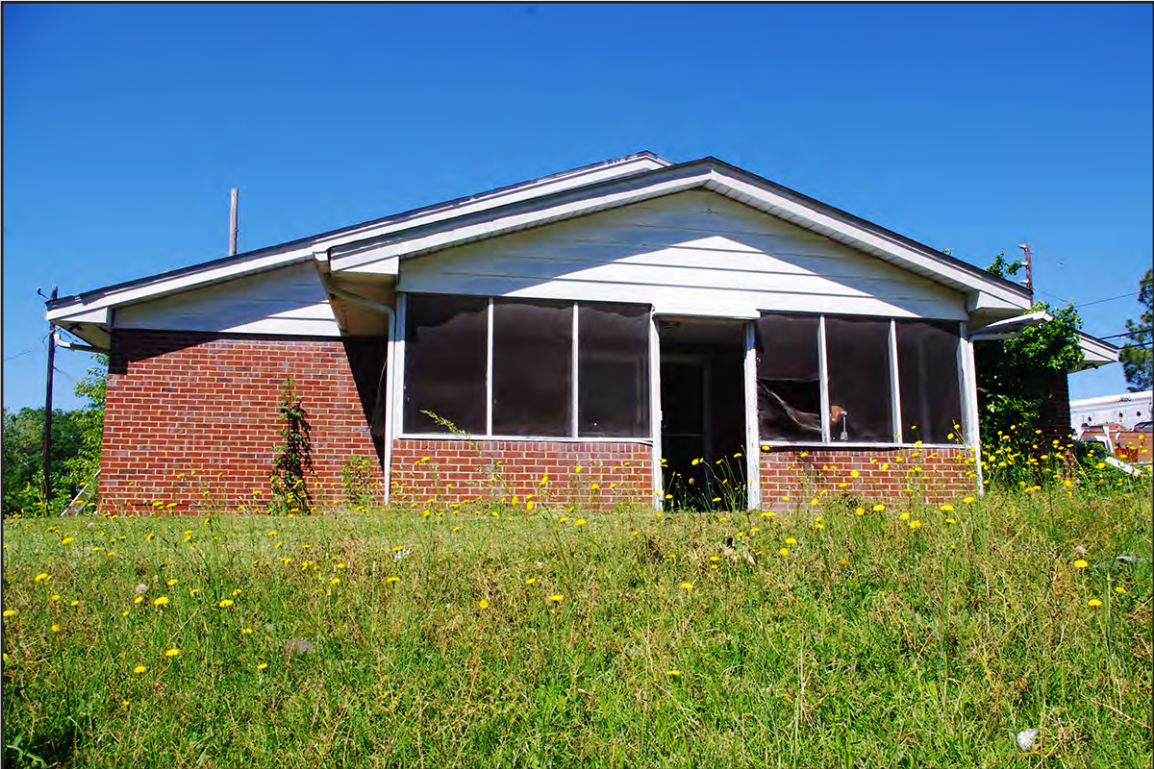
PLATE 22: Glenwood Rest Home (County Home) (RH0667) Annex, East Elevation, Rockingham, North Carolina
