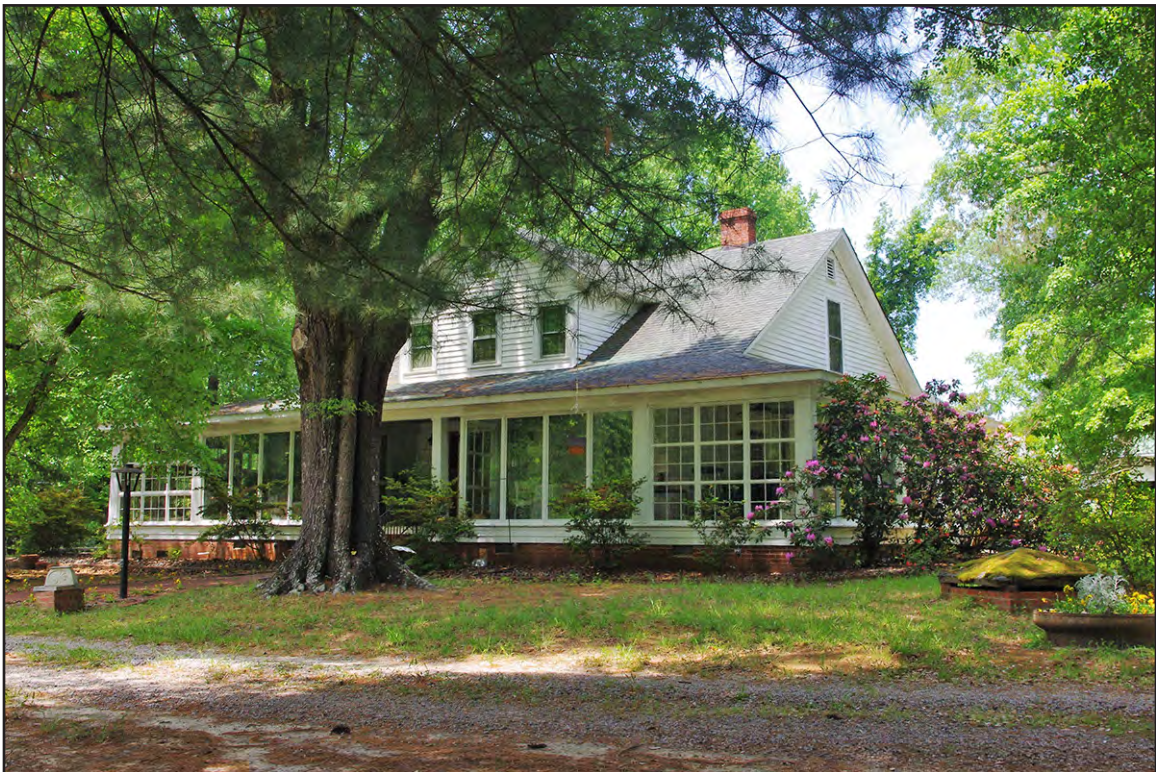
PLATE 70: Elliot-Terry-Mossor House (RH0297), Oblique View of East Elevation, Rockingham, North Carolina
