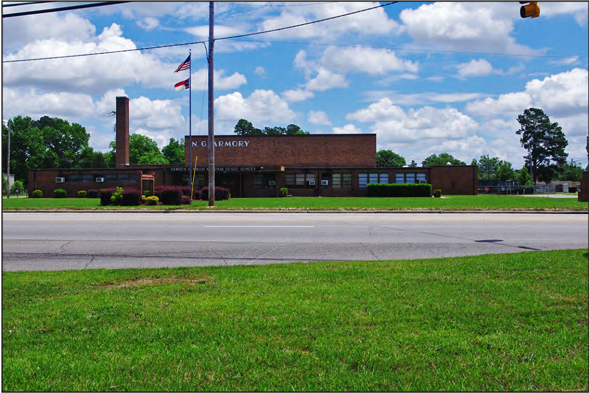
PLATE 8: Laurinburg National Guard Armory (SC0362), West Elevation, Scotland County, North Carolina
