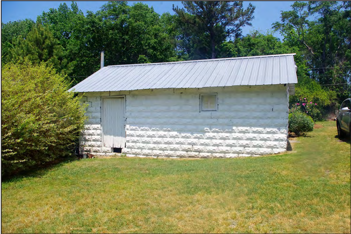
PLATE 115: Storage Outbuilding, South Elevation, Gibson-McDonald House (RH0156), Rockingham, North Carolina
