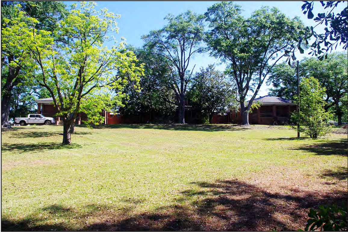
PLATE 11: Glenwood Rest Home (County Home) (RH0667), South Elevation, Rockingham, North Carolina
